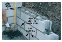
Build the ends of the wall Set out the first course of blocks, laying them out dry on the footing, ensuring the corners are square. Mix the mortar and lay the blocks. Build the end or corner with block centres over the joins of the course below.
